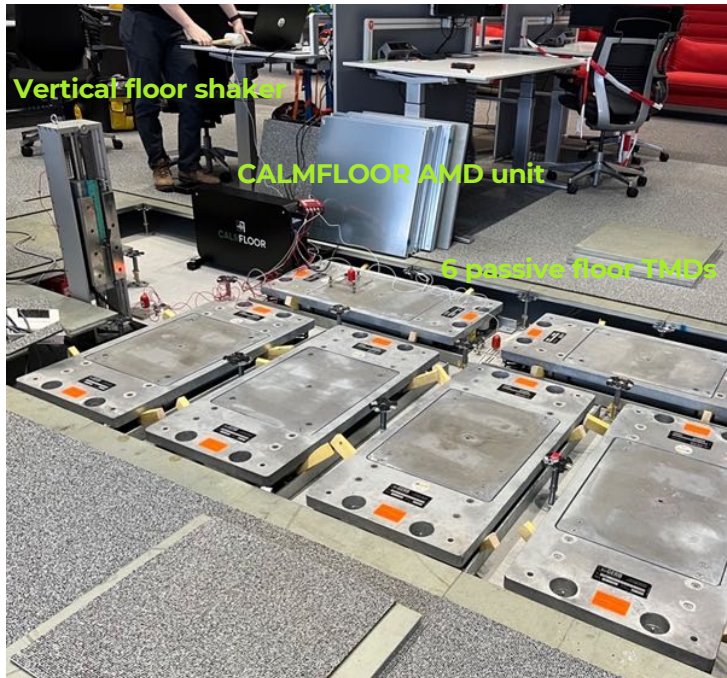
Figure 2: Six TMDs each with 250 kg moving mass and one 67 kg CALMFLOOR demo unit on top of the structural floor.
